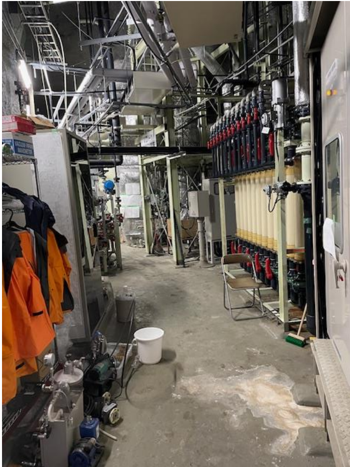
Super-K water cleaning plant
