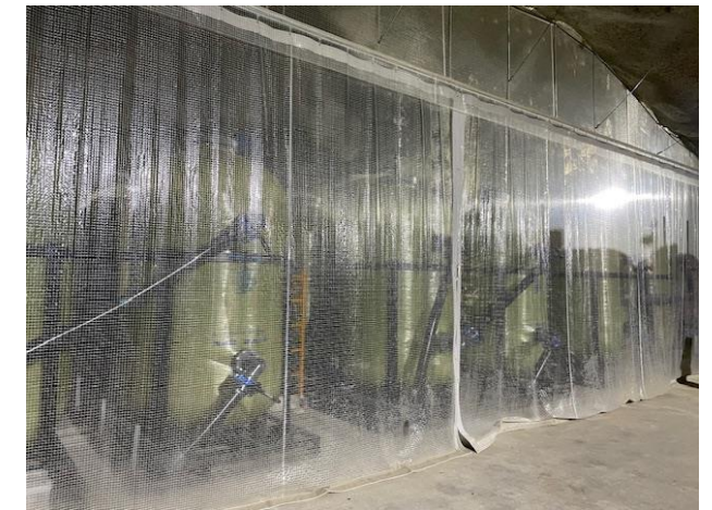
Hypr-K Gadolinium sulphate storage (top) and dissolution plant (bottom)
