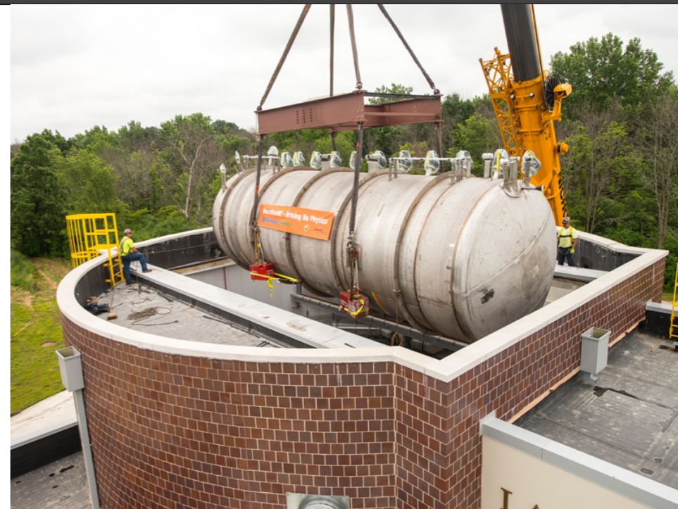
MicroBooNE cryostat lowered into the pit
