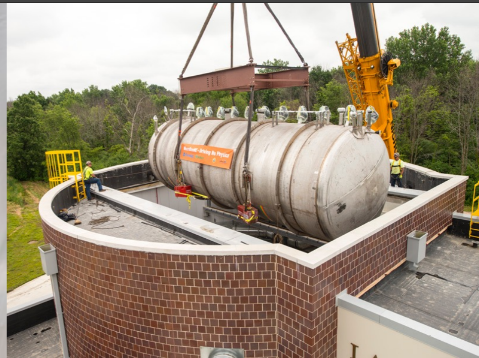
MicroBooNE cryostat lowered into the pit
