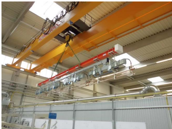
Waveguides at girder during installation test
