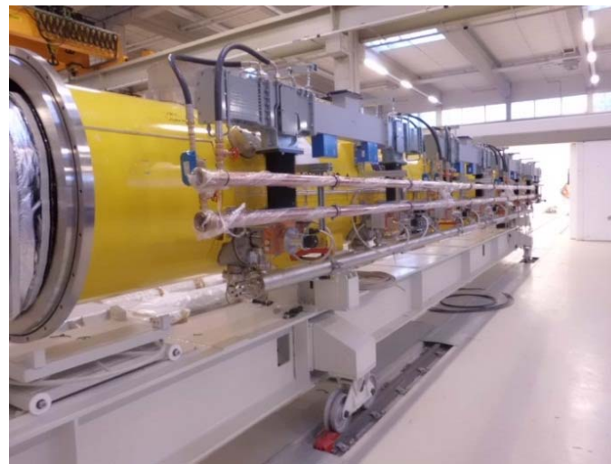
Waveguides with cooling tubes at module during installation test
