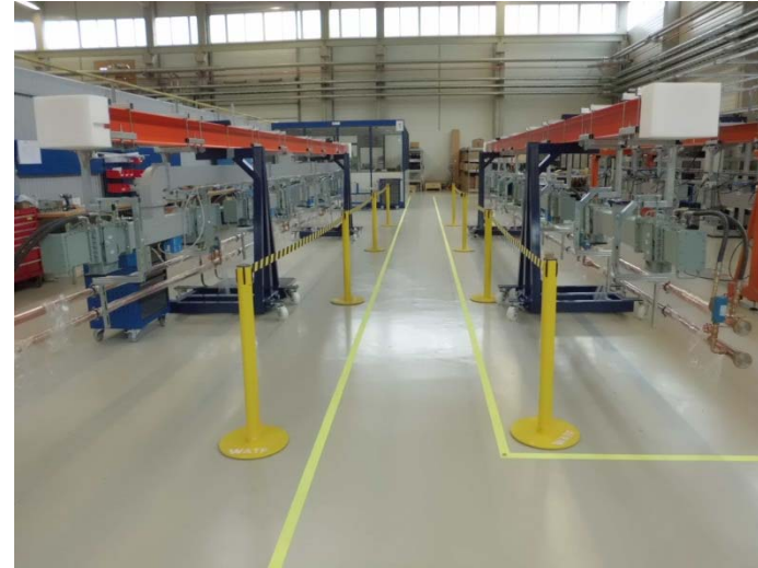
WATF with girders for waveguide assembly
