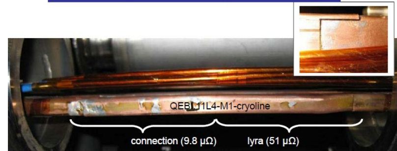
Sector 3-4 : QEBI.11L4-M1-cryoline before repair
